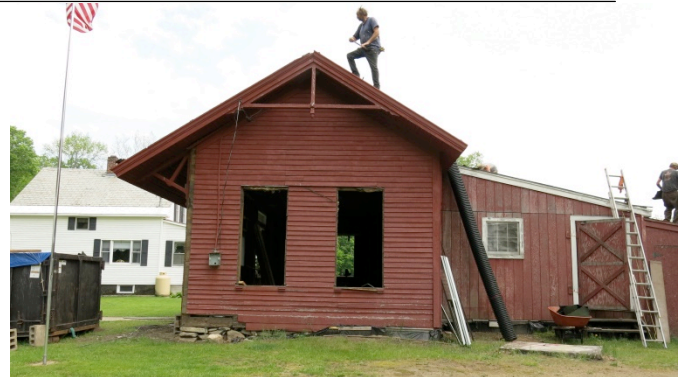
Deconstructing the Townshend RR Depot
