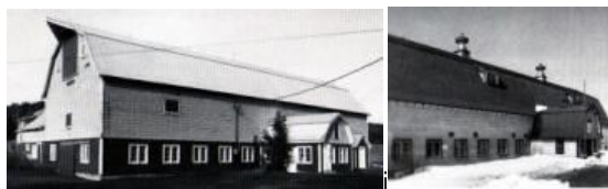
Ground-Level Stable Barns: Images courtesy of Thomas Visser.
