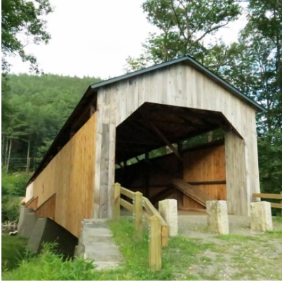
Scott Bridge, west bank.
